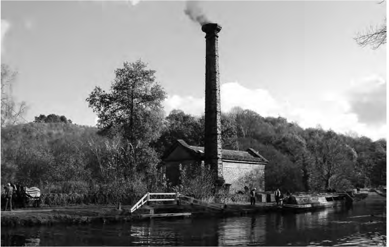
Leewood Pumphouse on the Cromford Canal
