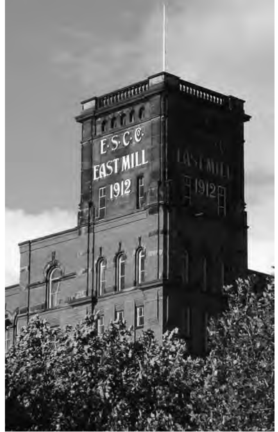
Belper's East Mill water tower
