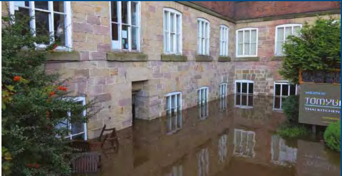
Flooding at the Belper Mill Complex, 2019
